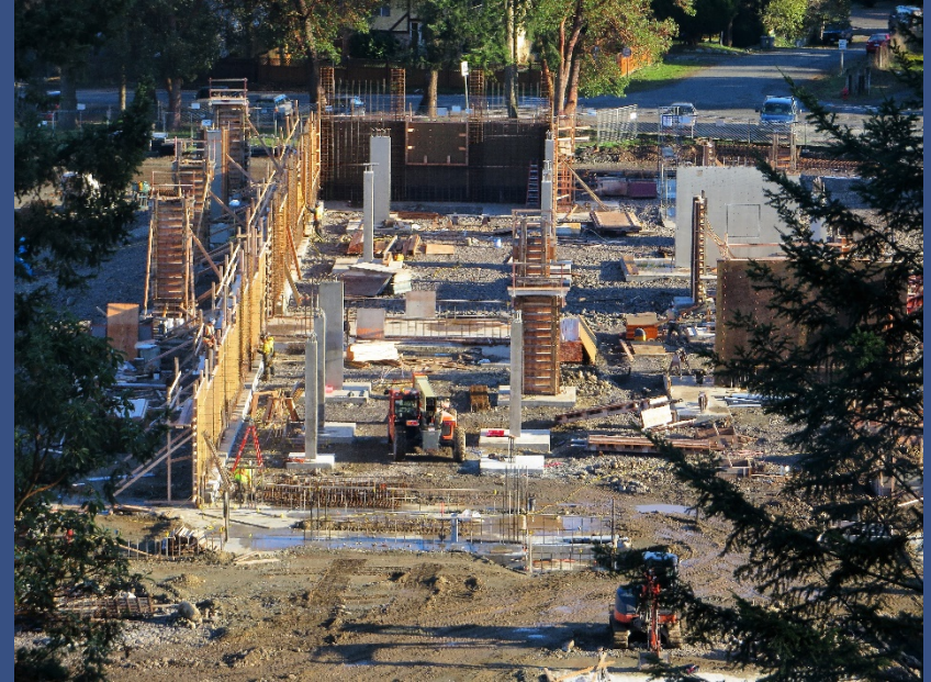
Construction of the new building on Langford Lake Road.
