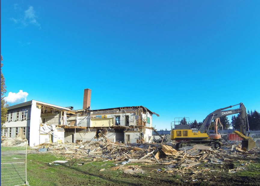
A bulldozer cleans up debris from the south end of the Jacklin Road old building.
