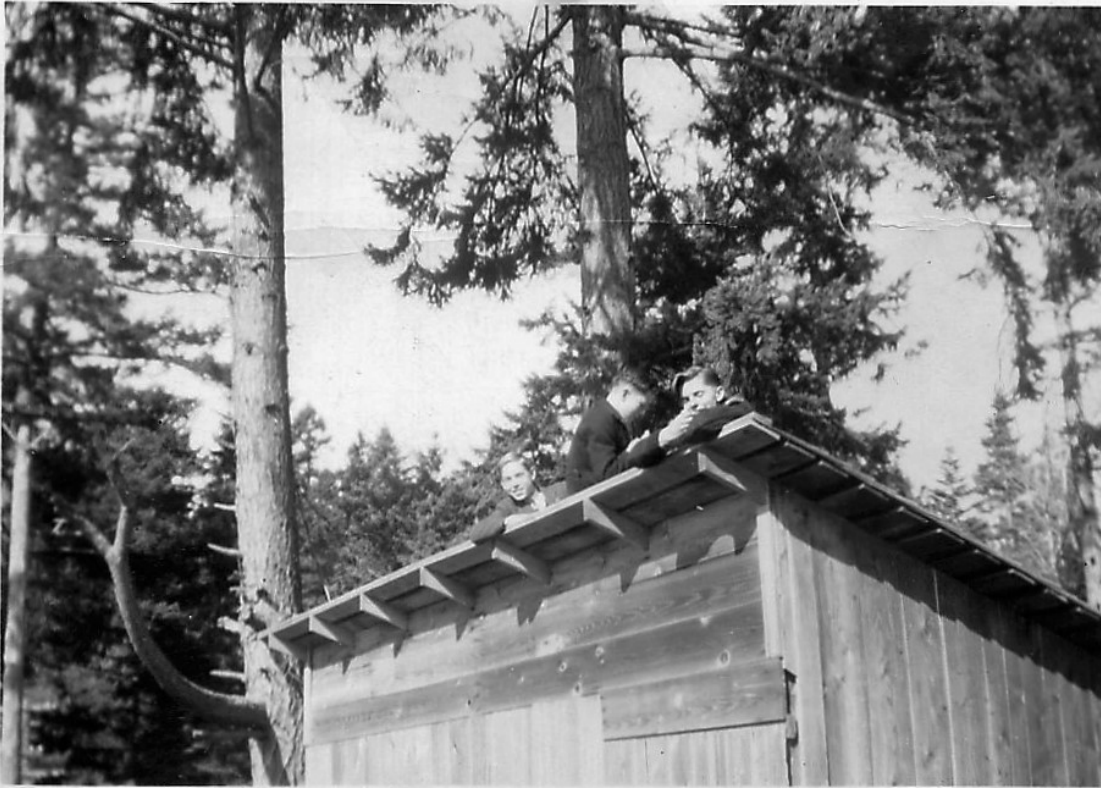
Tom Howard, Barry Lucas and Dale Absolan on the outhouse roof
