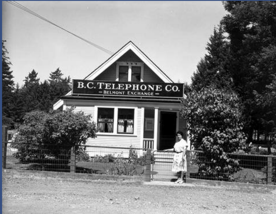
Belmont Telephone Exchange (photo from John James on the Old Victoria site)
